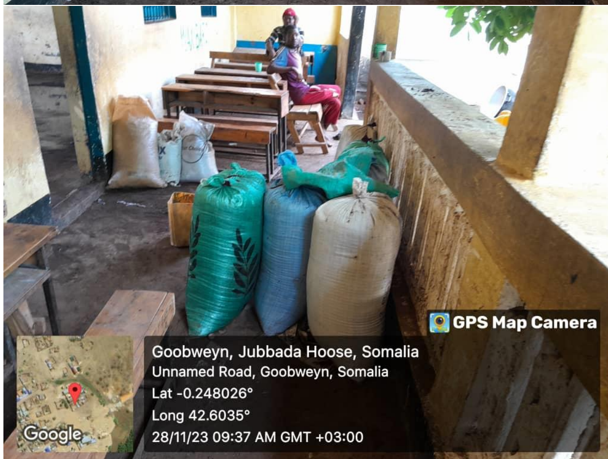
Some of the classrooms in Gobweyn Primary School used as a shelter by the displaced persons
